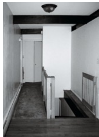
Skylights were installed in the upstairs hallway and the master bath and closet to brighten windowless areas.
